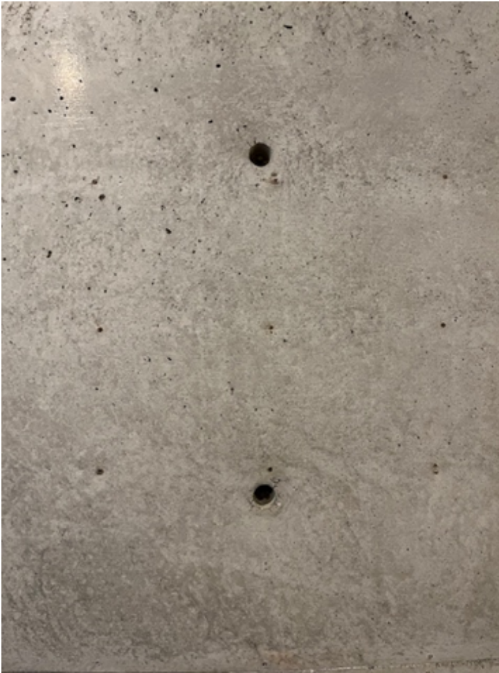
Detail of Fair-Faced Concrete Wall with Tie Holes Benesse House Museum
