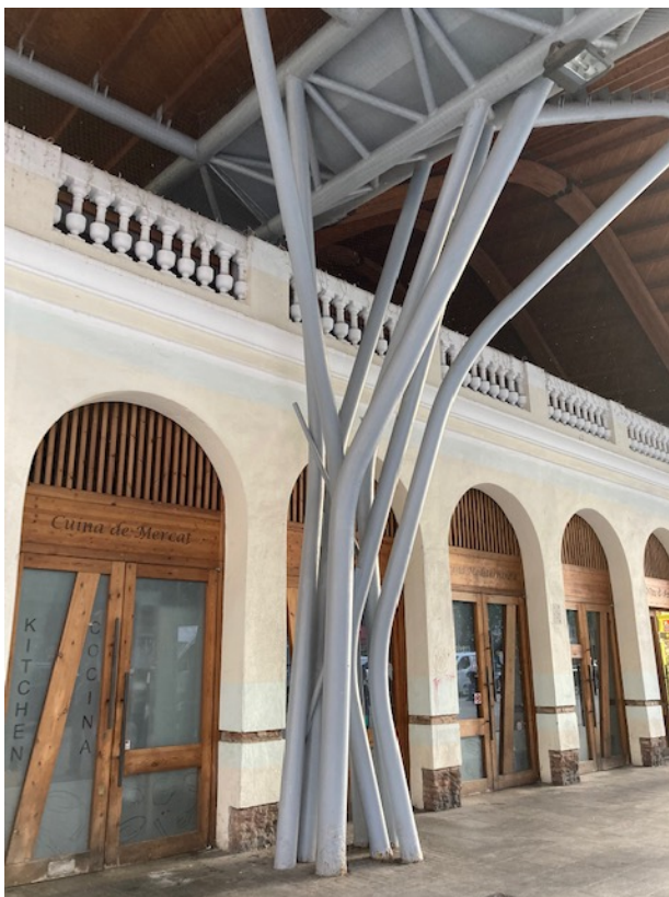
Santa Caterina Market Renovation Barcelona, Spain (2005)
